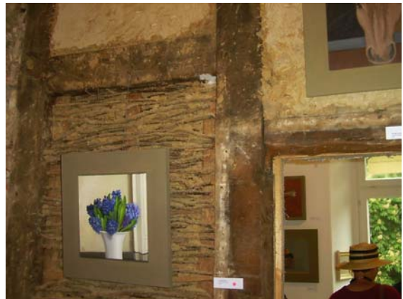
Building Construction. Fig. 2 Wattle and daub wall old German house, now used for exhibitions (photo by the author).
